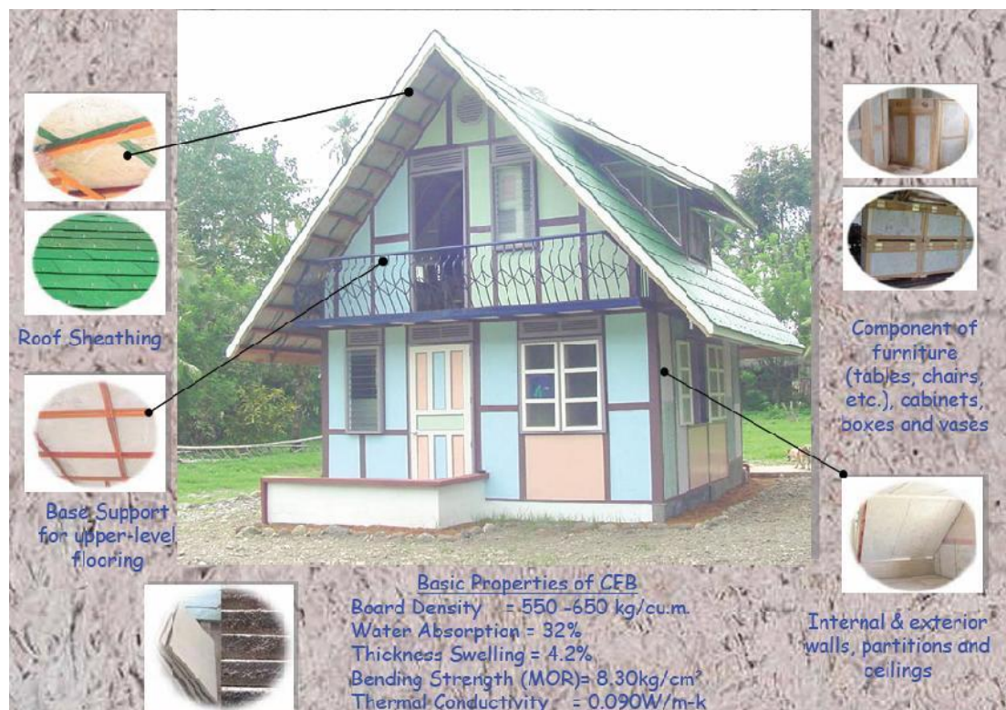
Fig. 4. Applications of Coconut Fibre Boards in House Construction and Other Utilities [Luisito et al. (2005)]
