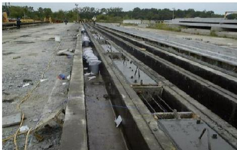
**FIGURE 2** Cylinders and Finished Piles with Embedded Shrinkage Plates
