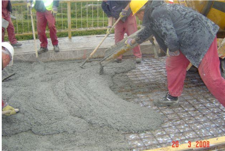
Fig. 5. Concrete placement during the bridge deck repair work
