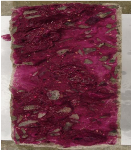
Fig. 6. Concrete Test Cylinder Showing Depth of Carbonation
