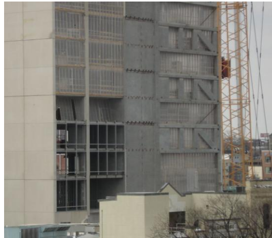
Fig 6: Precast Truss Erection
