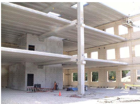
Fig. 4 Precast Example Structure 1, Plank Beams, Columns
