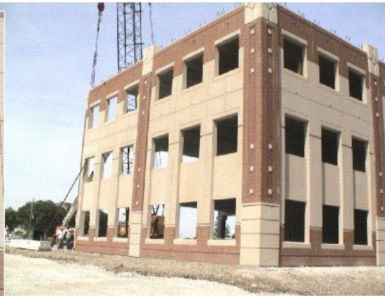
Fig. 3 Precast Example Structure 1
