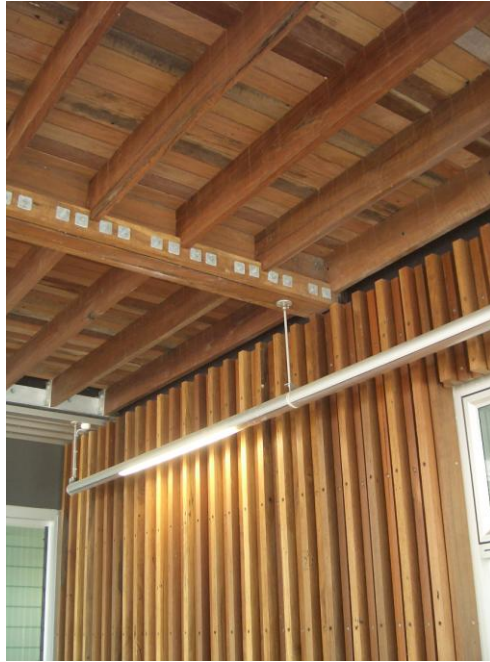
Fig. 2 Structural and decorative recycled Australian hardwood.
