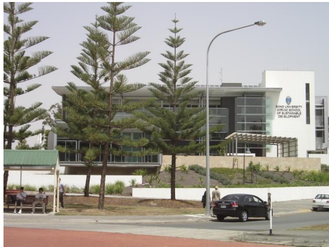
Fig. 1 The Mirvac School of Sustainable Development at Bond University, Queensland, Australia.
