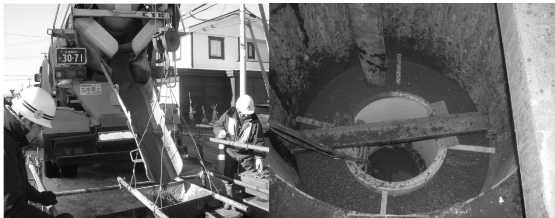
Fig. 13. Schematical view of backfill construction
