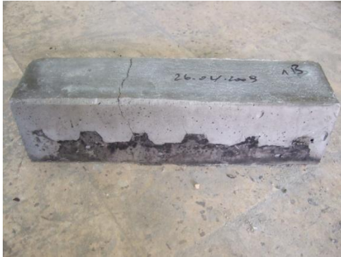
Fig. 2. A typical specimen with cracked overlay after demolding
