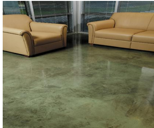
Figure 13. Ultra Thin Micro Topping with Waterbase Stain.
