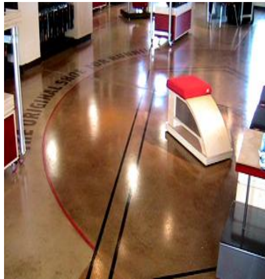
Figure 8. Acid Stain in Retail Area
