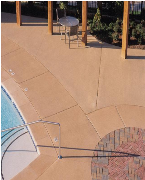
Figure 9. Integral Colored Concrete Hotel pool deck.
