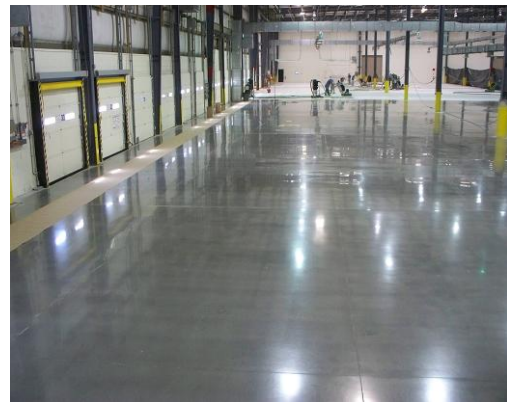
Figure 19. Commercial Warehouse Waterburg, Vermont
