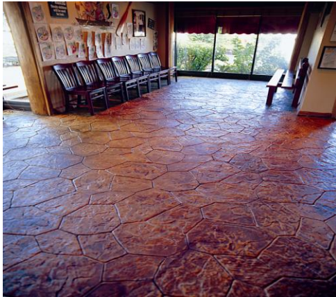
Figure 12. Thin Topping Material (3/16") Imprinted and Stained.
