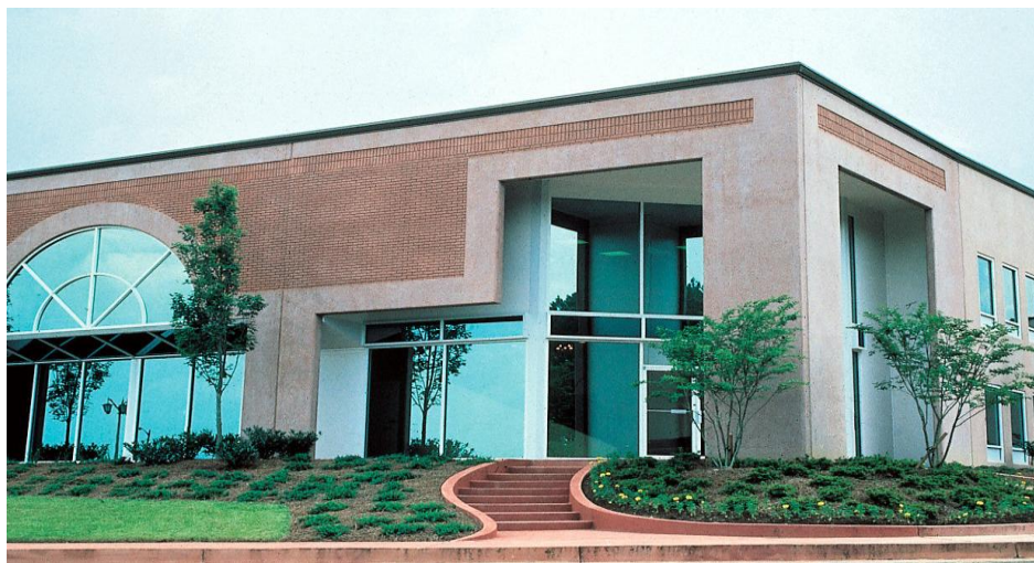
Figure 16. Tilt Wall project utilizing concrete for color and texture. Atlanta, Georgia. Headquarters, L. M. Scofield Company
