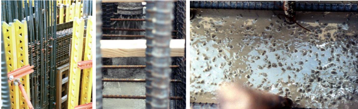
Fig.15-17 Dense reinforcement necessitated self consolidating high performance concrete.
