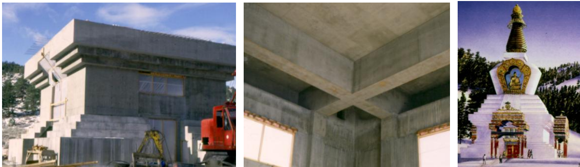
Fig.29-31 A 1000 year concrete design for the Great Stupa of Dharmakaya, Ft.Collins Colorado
