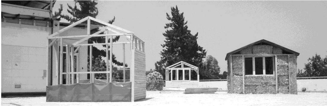
Fig. 5. Construction of physical test chambers, progress January 2010
