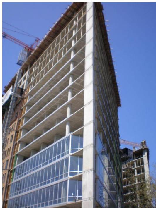
Fig. 4 Park Lafayette Construction.
