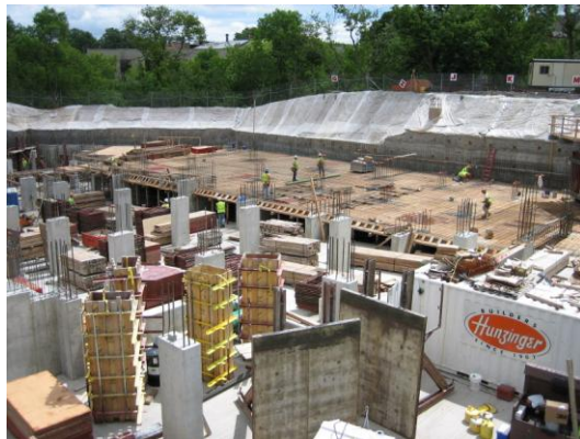
Fig. 5 Park Lafayette Construction
