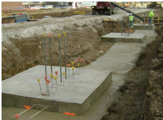
Fig. 1. Johnson Controls Footings and Flowable Fill
