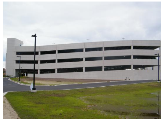
Fig. 2 Johnson Controls Precast parking structure
