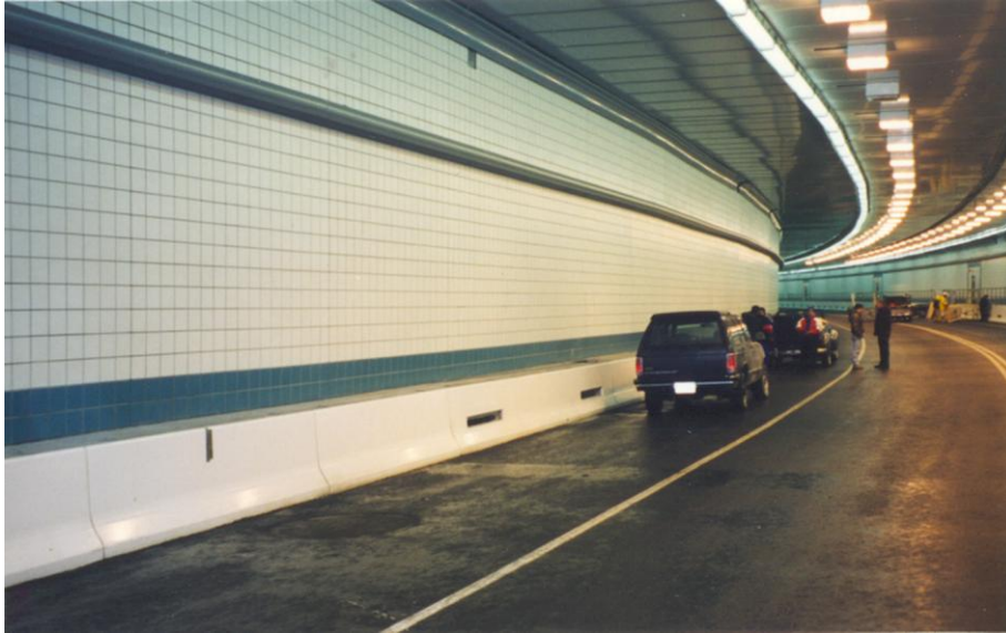
Fig 4. Precast Polymer Concrete panels used for tunnel bench wall.
