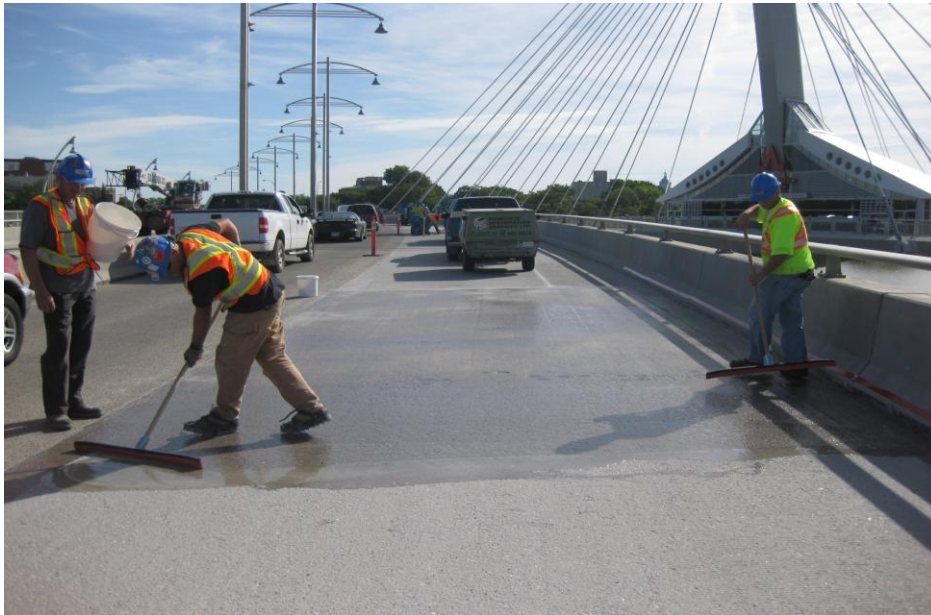
Fig 1. HMWM Resin brushed/squeegeed onto bridge deck.
