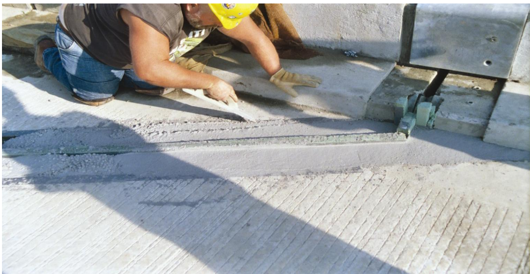
Fig. 2 MMA Polymer Concrete for a Bridge Expansion Joint/Header
