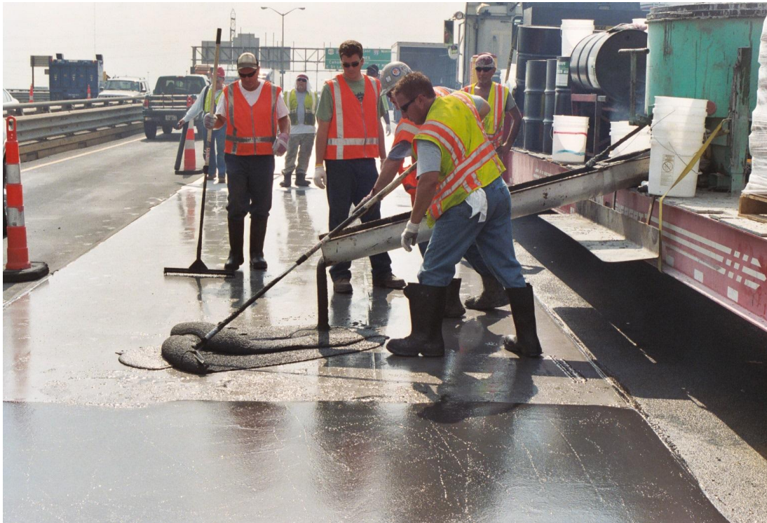
Fig 3. MMA Slurry Overlay spread with gauge rakes.
