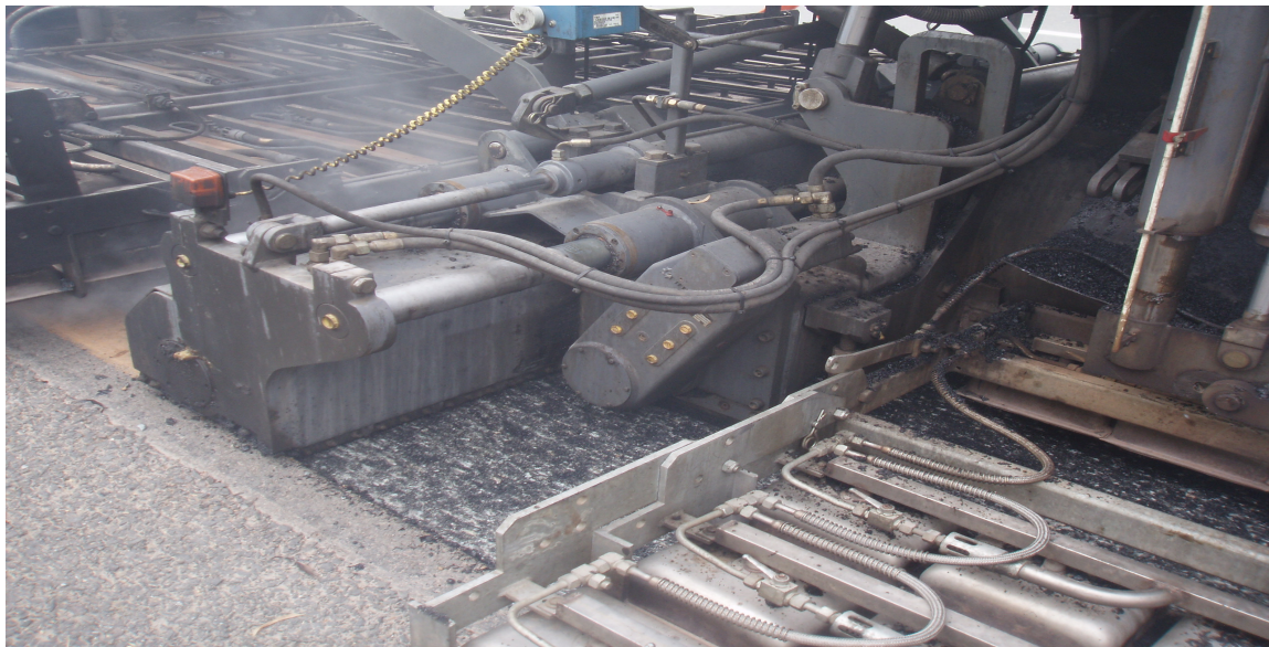
FIGURE 6 Scarifying and heating unit.
