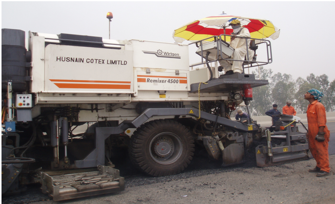
FIGURE 7 Remixing unit.
