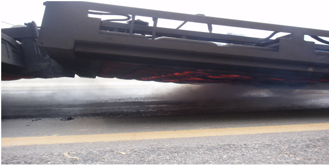
FIGURE 5 Pre-heating unit.
