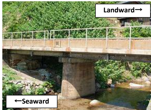
Figure 1. A picture of railway bridge
