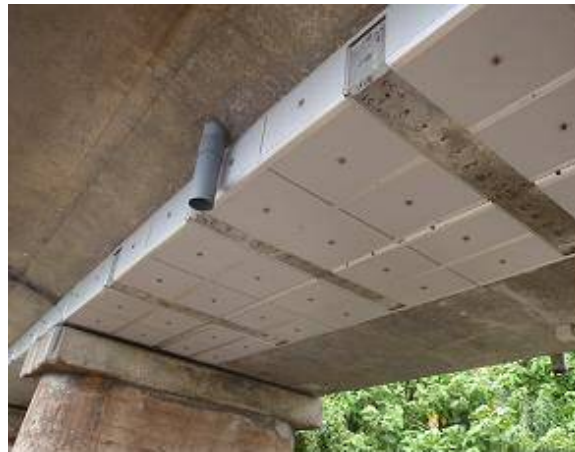
Figure 5. A picture of Aluminum panels at railway bridge
