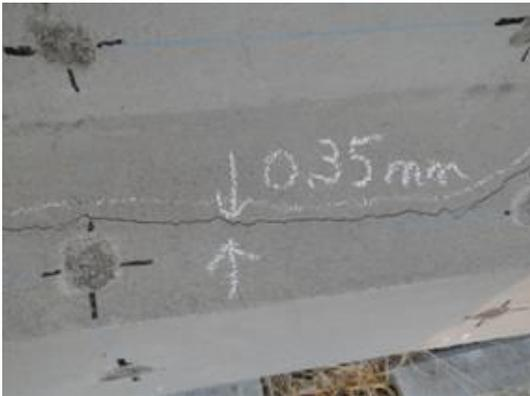
**Photograph 1. Crack of Over-lay Mortar (TM system : normal protective)**
