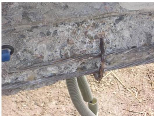
**Photograph 2. Corrosion Condition of PC Wire (TG system : after 10 year)**
