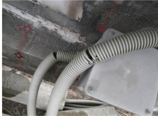
**Photograph. 4 Condition of Pipes (after 10 years)**
