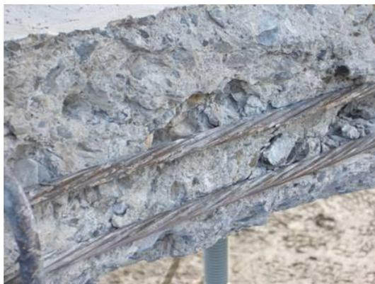
**Photograph 3. Corrosion Condition of PC Wire (TM system : normal protective : after 10 year)**
