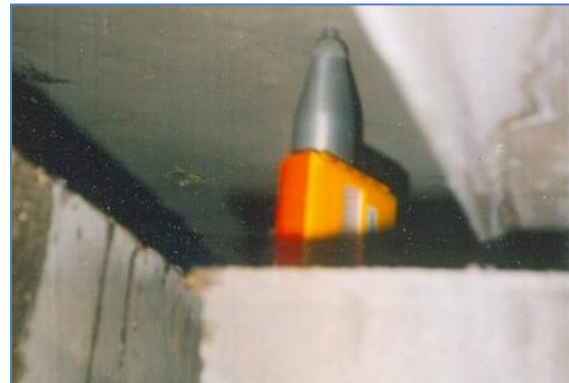
b) On Soffit of Bottom Slab
