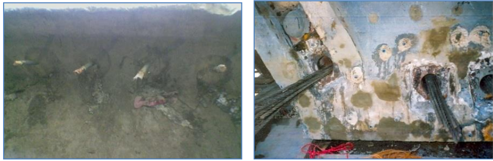
Figure 7. View of the Span after Repairs
