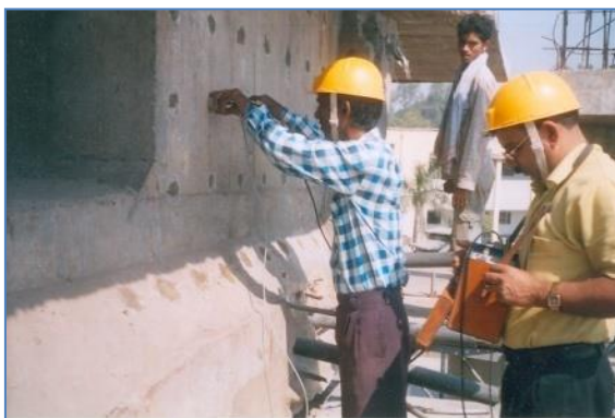
a) On Diaphragm Wall
