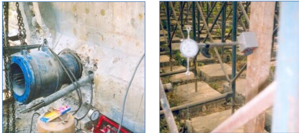
Figure 8. Deflection Measurements of the Span during Prestressing of Tendons
