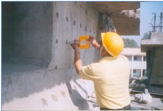
a) On Diaphragm Wall
