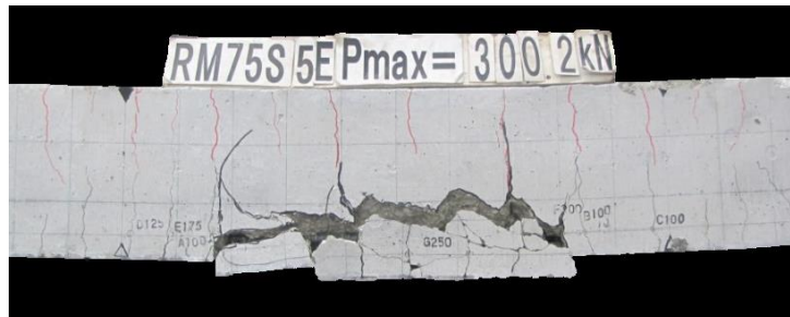
Figure 7. Final failure pattern for RM75S5E (Pure bending section)
