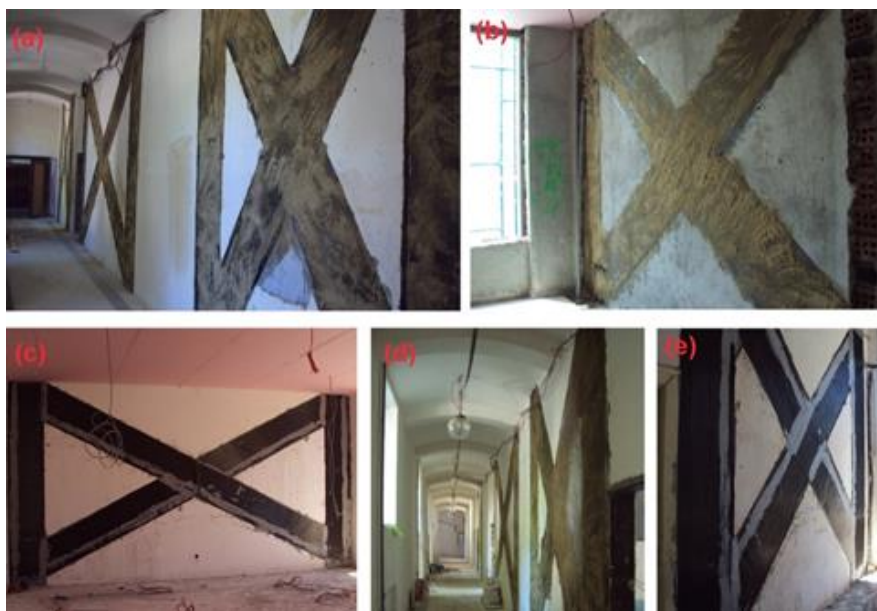
Figure 5. Retrofit applications made using CFRP wrap, (a-e)
