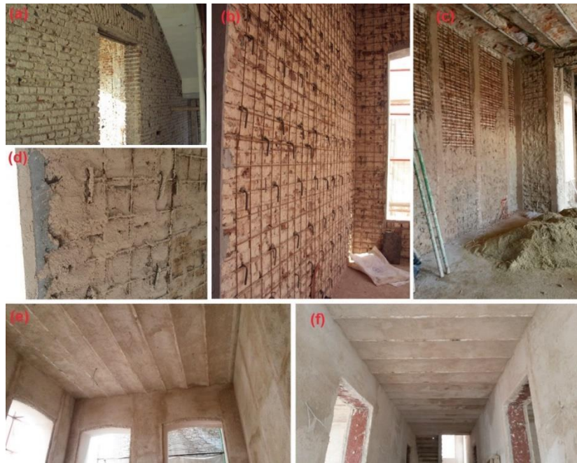
Figure 4. Strengthening plaster application stages, (a-f)
