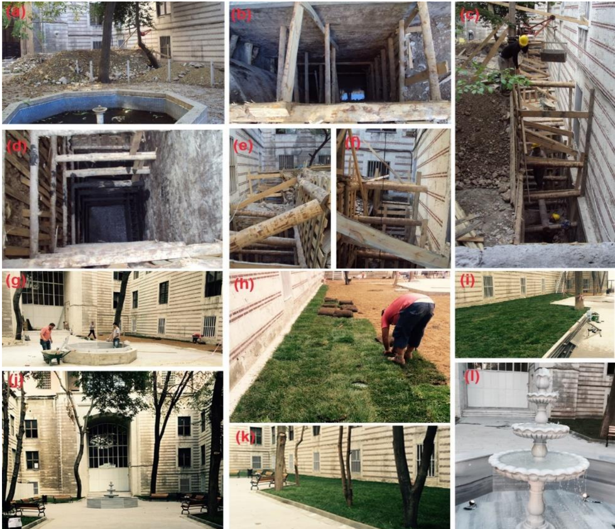
Figure 3. Well basis application and landscaping applications, (a-l)
