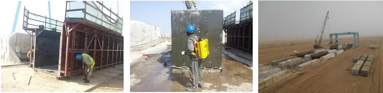
**Figure 2. Mass Concrete Blocks for the Wharves at Jizan Seaport**
