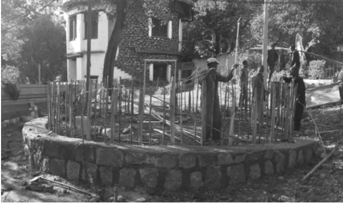
Fig 3. Juniper tree poles used for foundation
