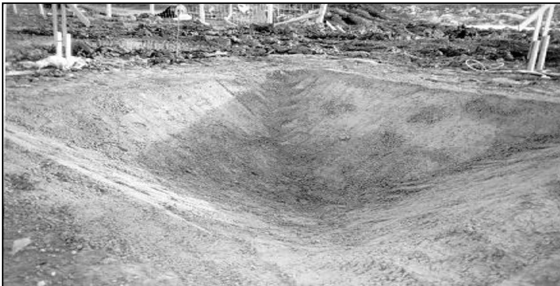
**Figure 4:** Finished landfill cell after compaction of spent borax concrete layer.
