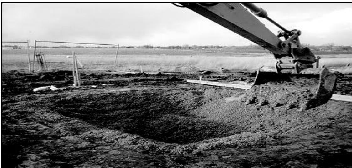
**Figure 3:** Emplacing the top layer spent borax concrete.
