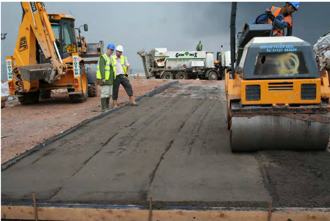
Figure 4. Compacting of the semi-dry paste layer using a 3-tonne roller
