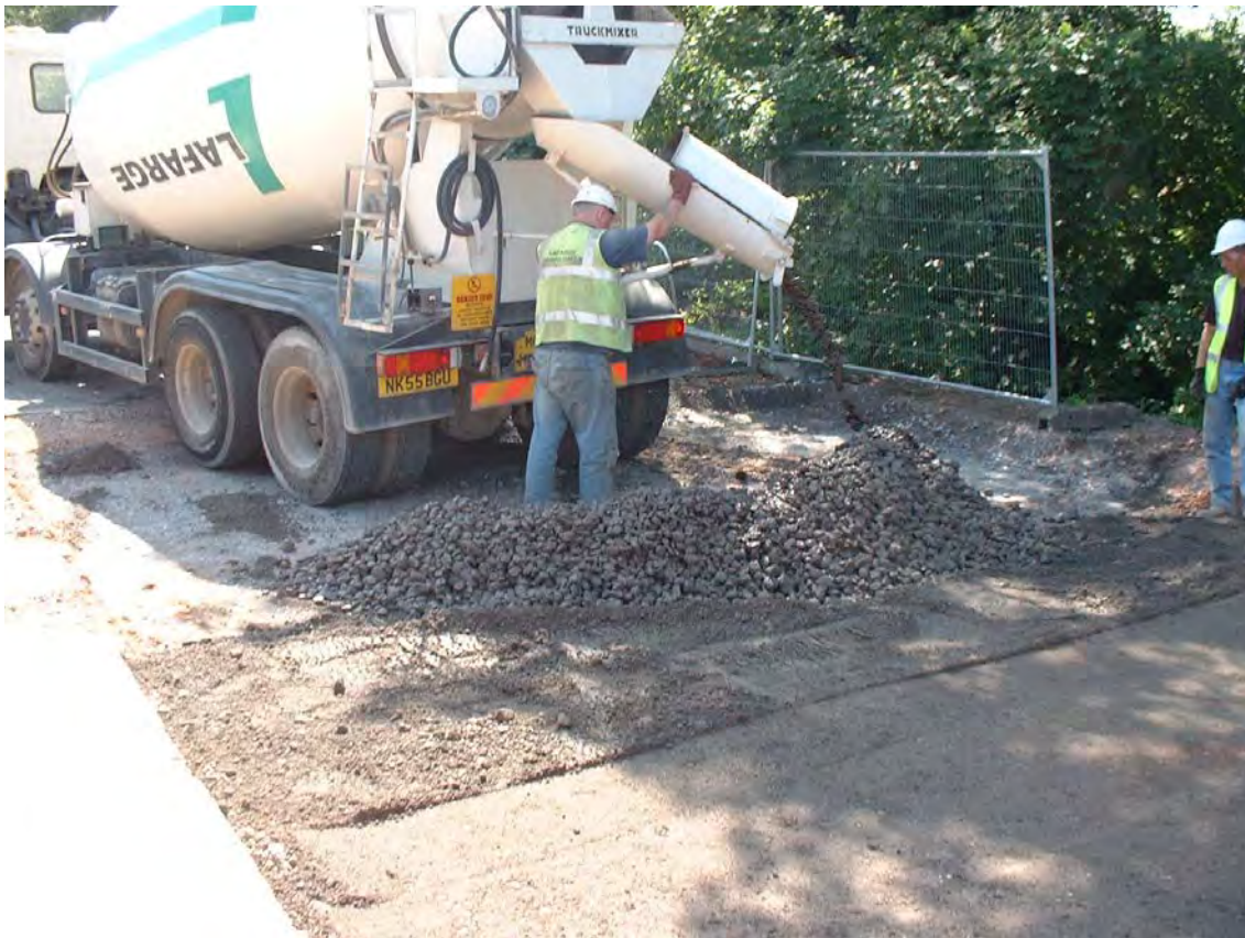
Figure 5. Placing and spreading the concrete
