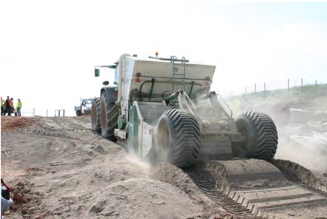
Figure 1. Blending the mixture of soil and binder using the rotavator
