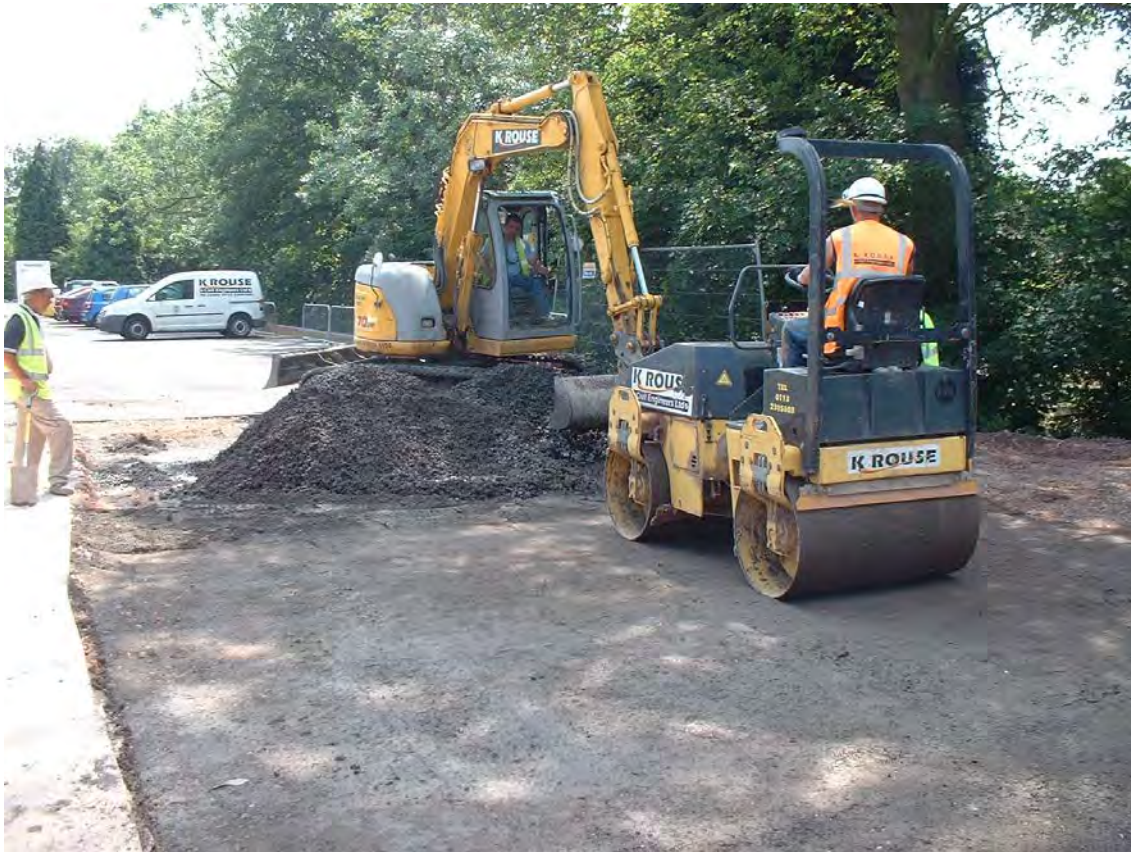
Figure 6. Concrete compaction using a 3-tonne vibrating roller
