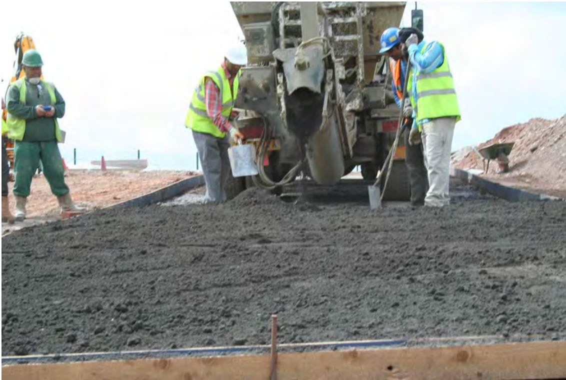
Figure 3. Spreading and levelling the semi-dry paste
