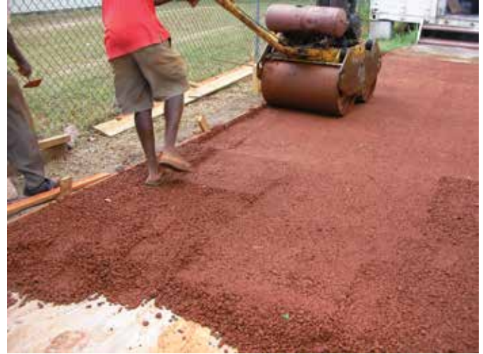
Fig. 3: Roller compacting the mixture
