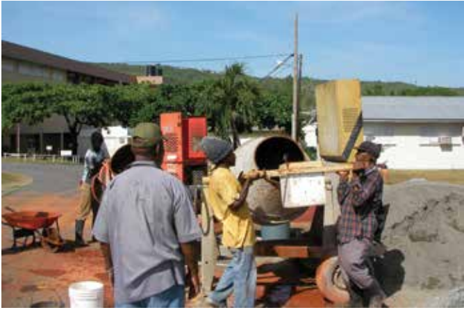
Fig. 2: Discharging a gauge box into the mixer
