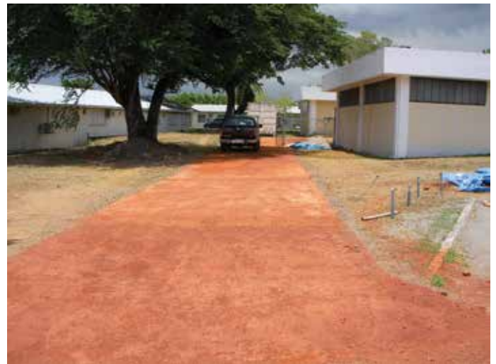
Fig. 4: The completed road
