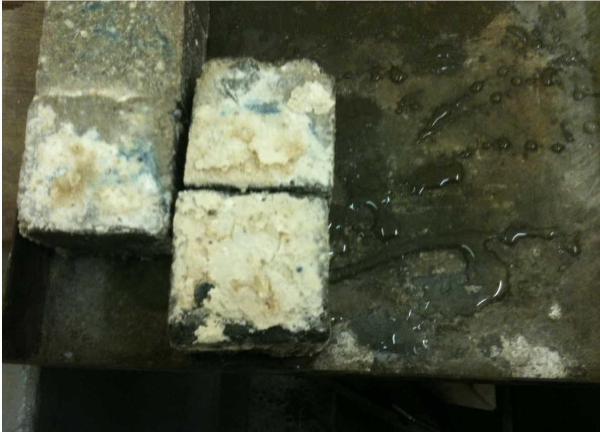
Figure 5.15: Lime Deposits on Binary Mixes - C
