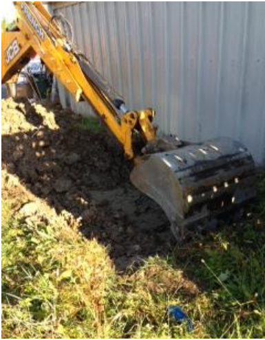
Figure 4.33 and 4.34: Excavation of Pit
