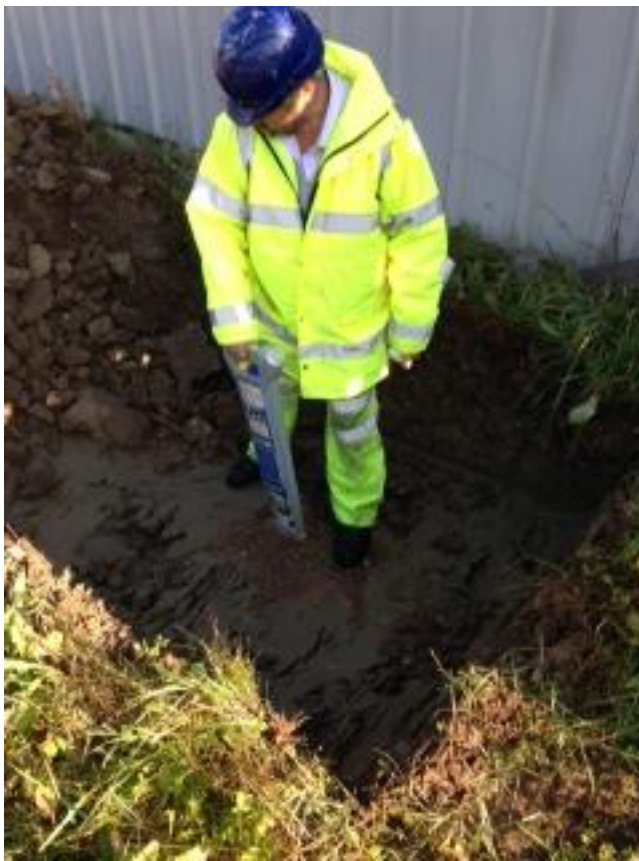
Figure 4.31 Detection of Underground Services
