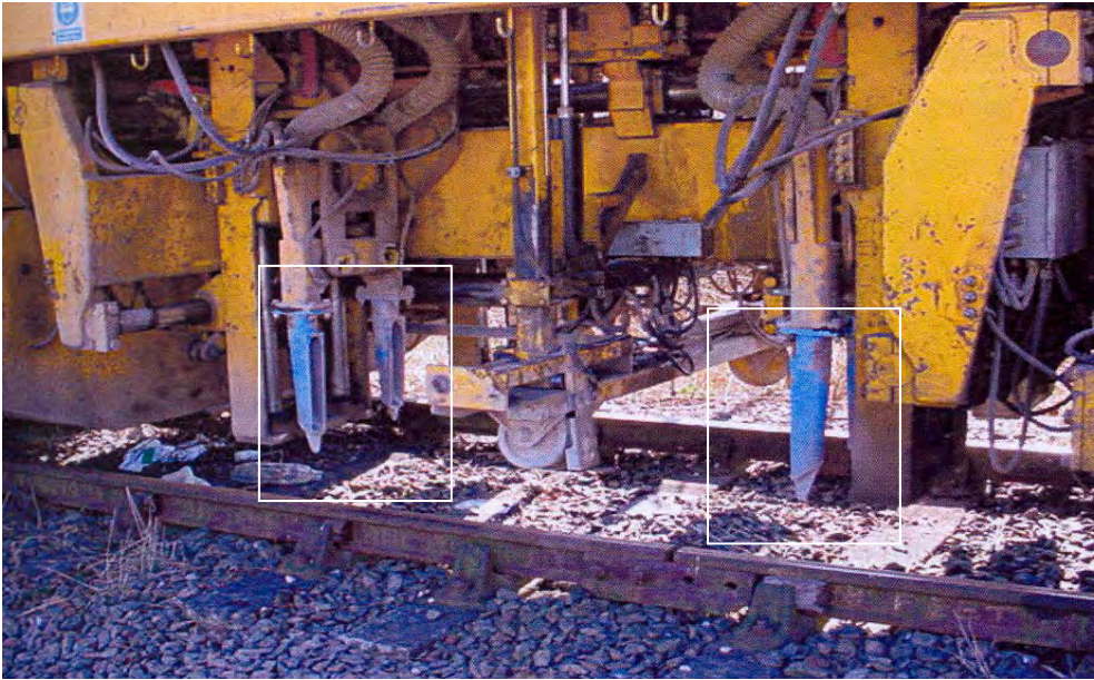
Figure 2.38 Close-up photograph showing the tubes used for blowing stones under the sleepers
