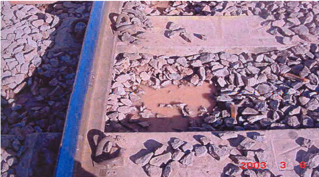
Figure 2.15 Wet spot with water ponding in the crib (Ball 2003)
