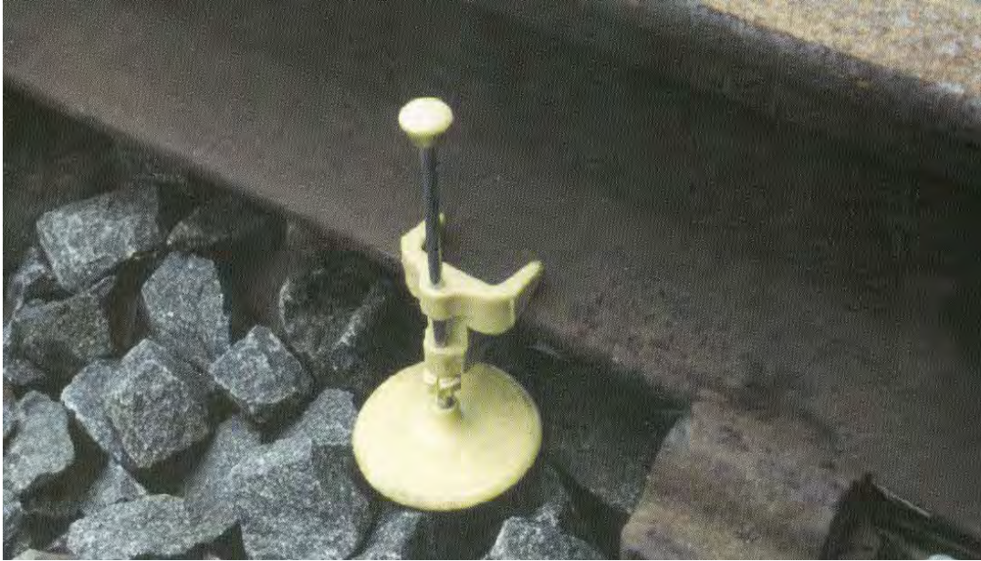
Figure 2.11 Showing Pell void meter fixed to bottom flange of the rail (Cope and Ellis 2001)
