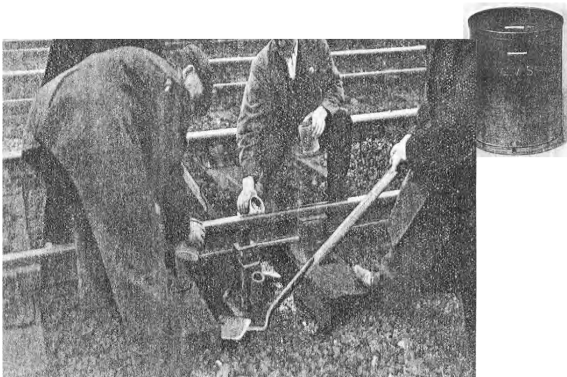
Figure 2.24 Measured shovel packing in progress, note the can used to measure the amount of chips required for packing (Fraser 1938)
