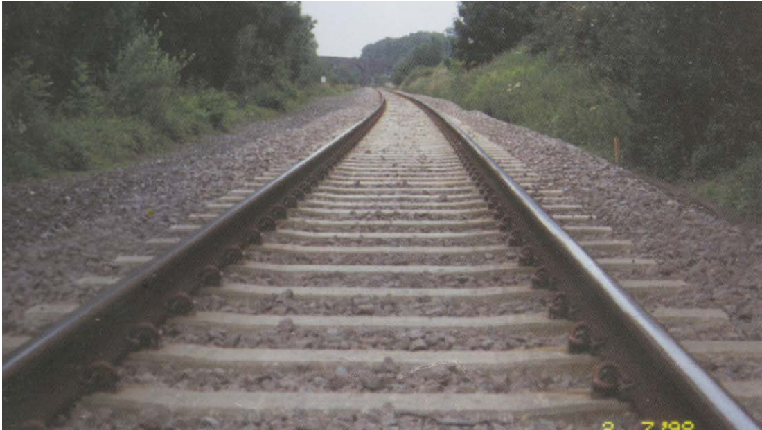
Figure 2.1 Ballasted railway track with concrete sleepers (Cope and Ellis 2001)
