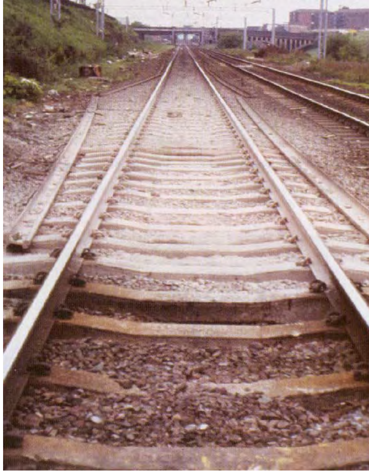
Figure 2.18 An advanced stage of wet spot which will require ballast renewal (Cope and Ellis 2001)
