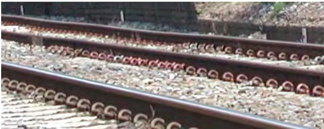
Figure 2.12a Coventry – Nuneaton railway line as seen from level crossing on Coundon Road in Coventry, close to the author’s house. Note the cyclic fault in the track. Speed limit of 35-40 mph is in force on the track as seen in the photograph.
