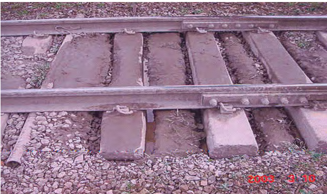
Figure 2.16 An advanced stage of wet with voided sleepers and fouled ballast (Ball 2003)
