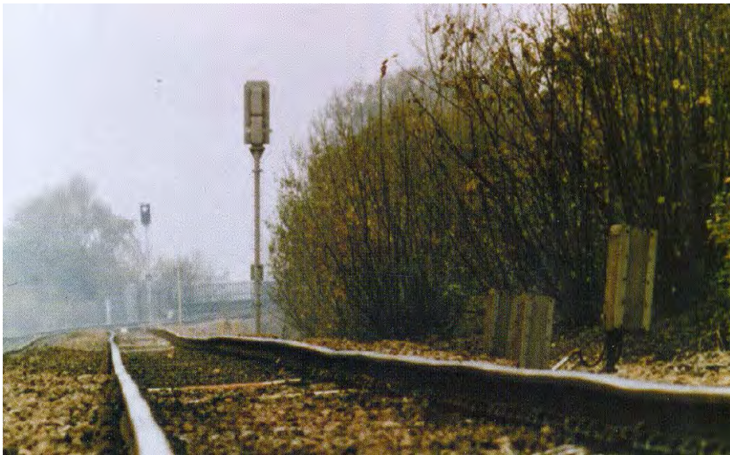
Figure 2.19 Cyclic top in continuous welded track. In extreme cases these dips can cause vehicle derailment (Cope and Ellis 2001)
