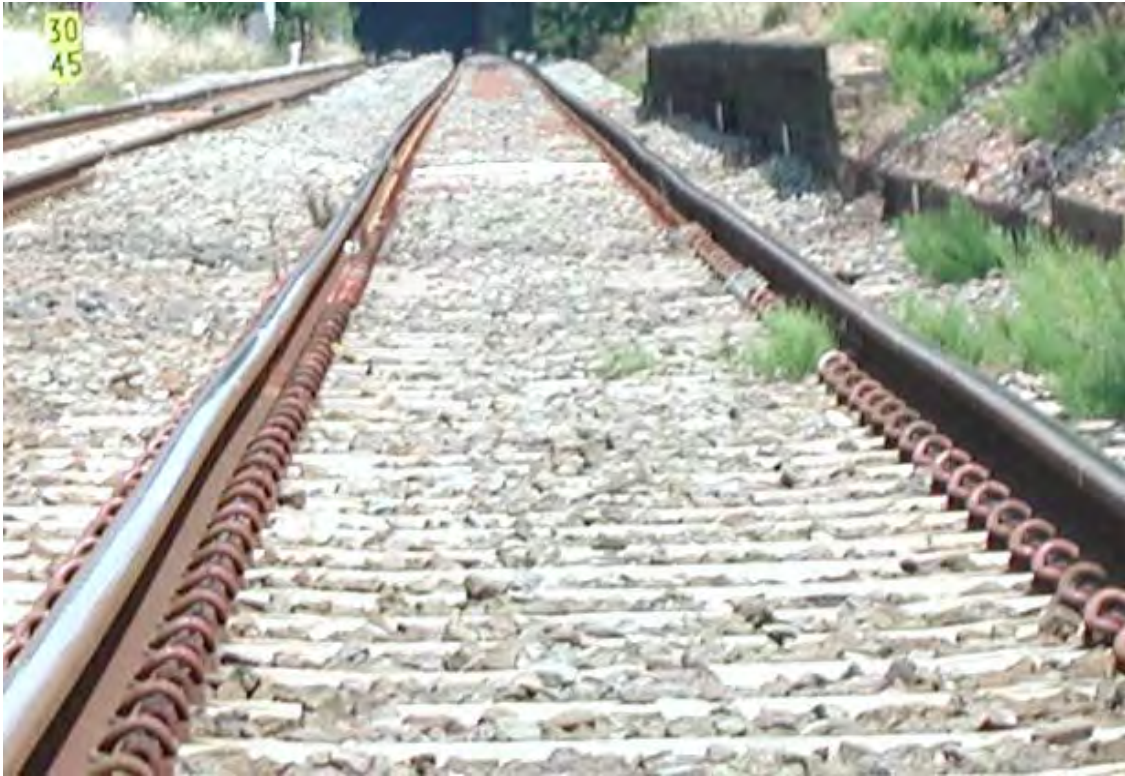
Figure 2.12a Coventry – Nuneaton railway line as seen from level crossing on Coundon Road in Coventry, close to the author’s house. Note the cyclic fault in the track. Speed limit of 35-40 mph is in force on the track as seen in the photograph.
