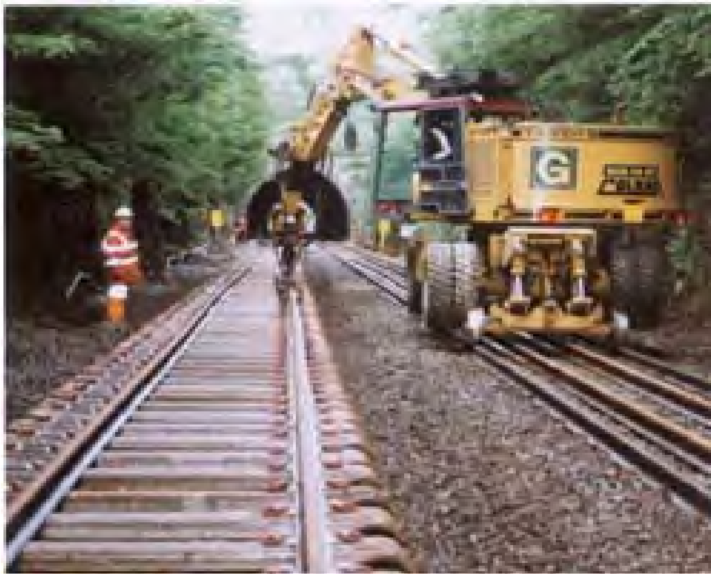
Figure 2.5 Track being laid on steel sleepers
