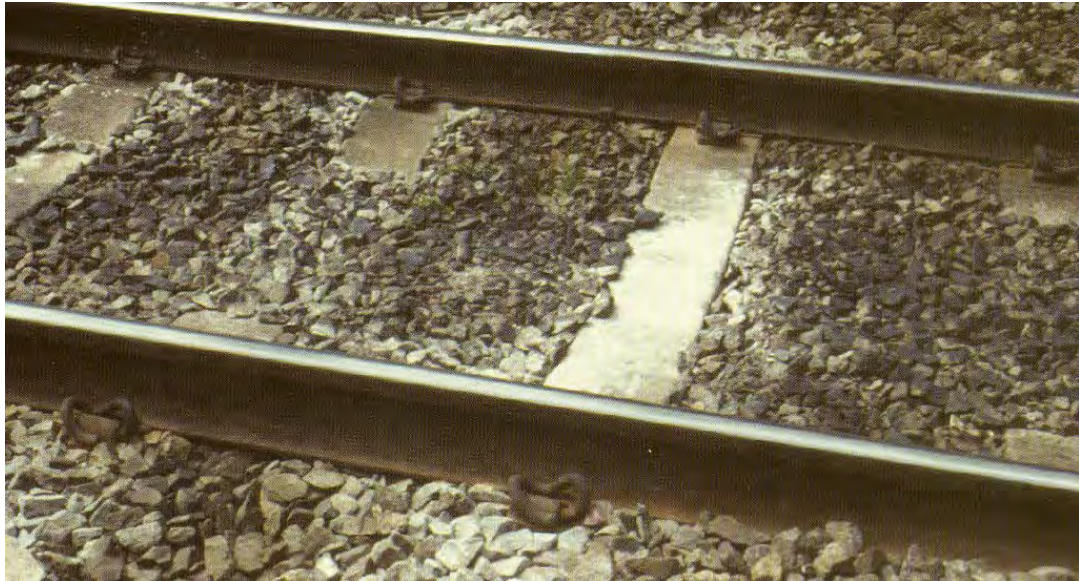
Figure 2.14 Voids below concrete sleeper again identified by white powder around the sleeper.
