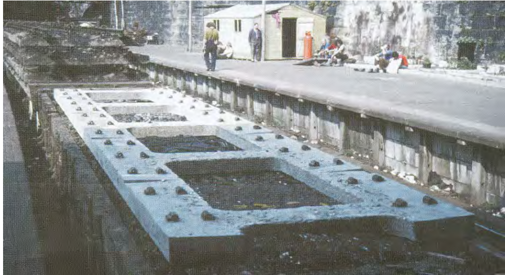
Figure 2.50 Ladder track used in the U.K.
