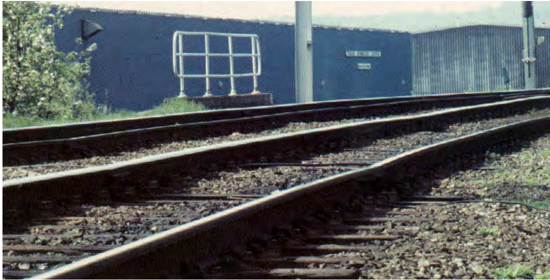
Figure 2.20 Dipped joints caused by insufficient packing of ballast below joints (Cope and Ellis 2001)
