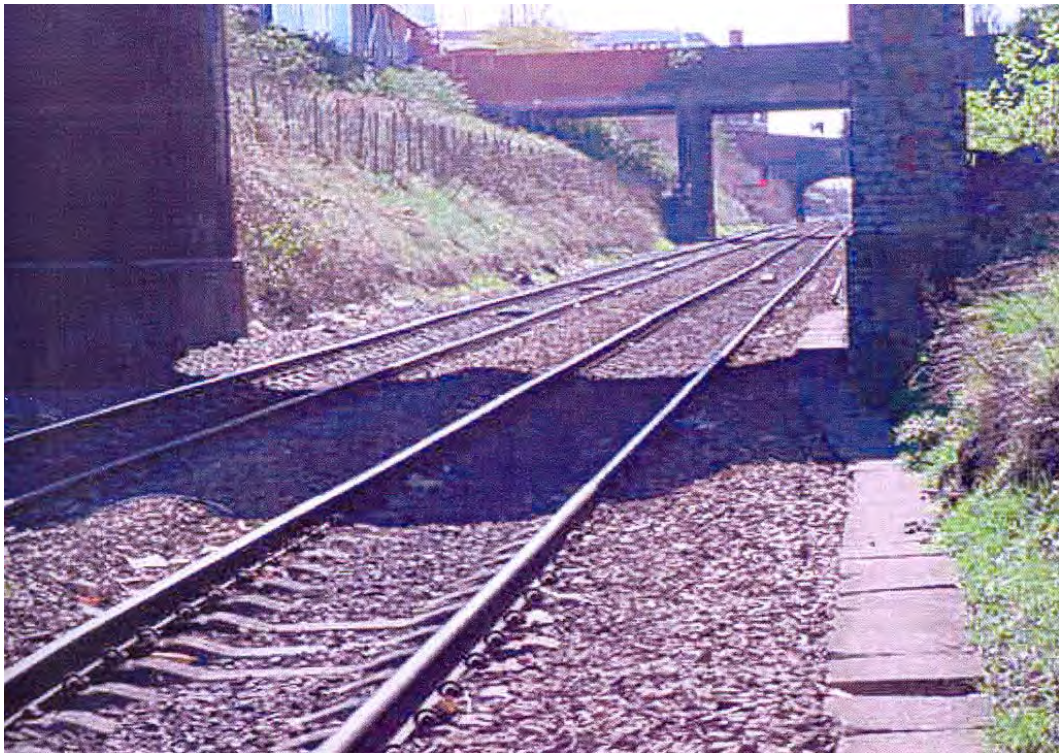
Figure 2.22b Track geometric quality restored by maintenance, standard deviation 3.1mm
