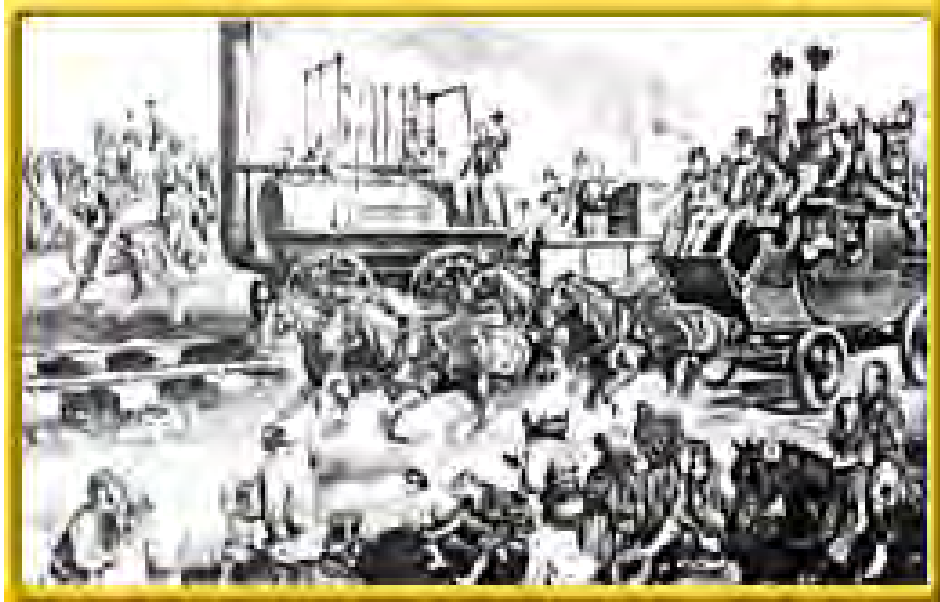
Figure 2.3 An artists impression showing the first passenger train ever run. It seems a horse drawn carriage was run alongside to compare the ‘horsepower’ of six horses to steam power but note the track in the foreground with rails sitting on top of massive stone blocks with no ballast ( www.railcentre.co.uk 2003)
