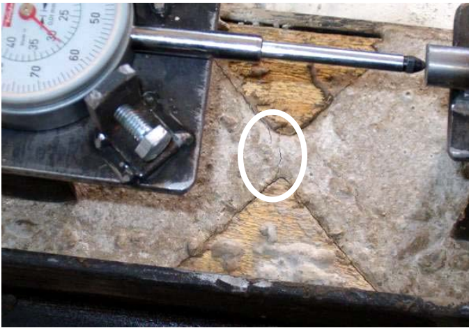
Figure 4. Particular of a shrinkage crack.
