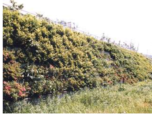
Figure 1. Revegetation area by leaning-type retaining walls (7 years after construction).
