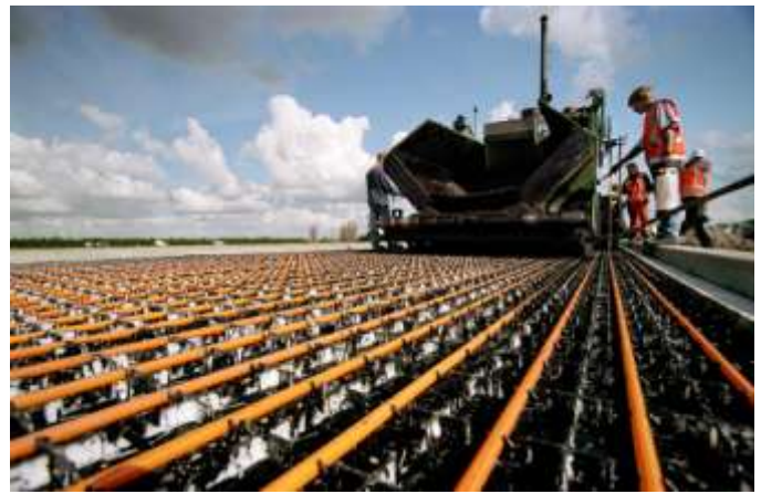
Figure 4. Overview of Final Asphalt Solar Collector System
